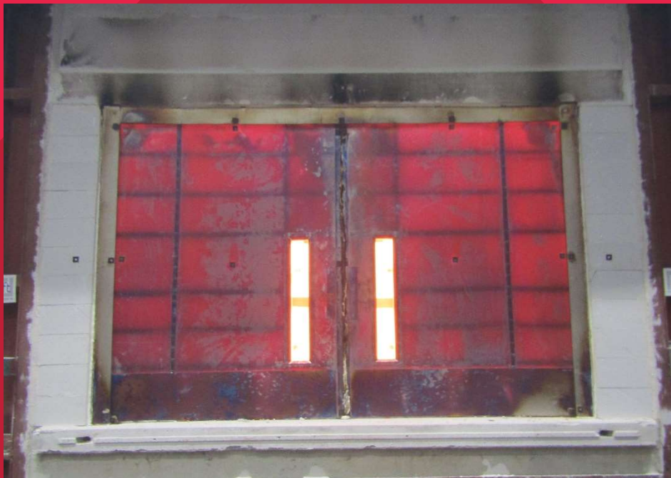
Successful completion of 100 minute fire test on 4.32m wide x 2.8m high double leaf test door
